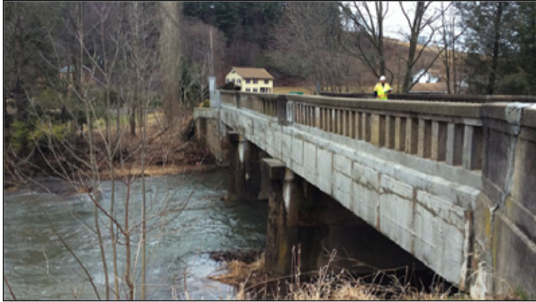
Fig. 1. Pennsylvania Rapid Bridge Replacement Project (Source: PennDOT).
