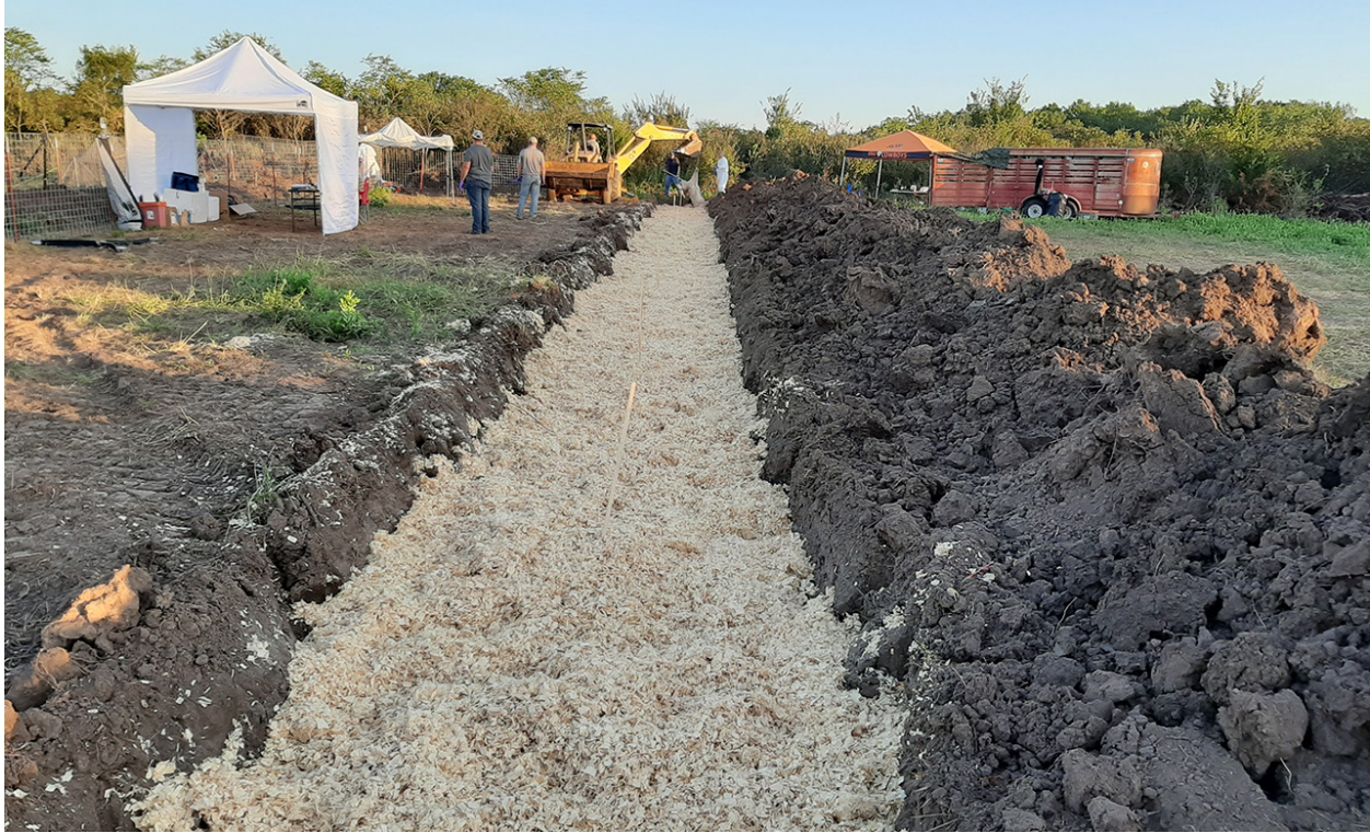
Fig. 4. Above Ground Burial trench prepared for the disposal of fifty 450-pound sows in Oklahoma in 2019 (Source: Gary Flory).
